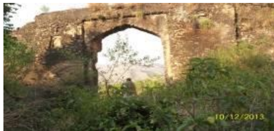
Fig. 21 View Ziarat Gate Pharwala Fort
