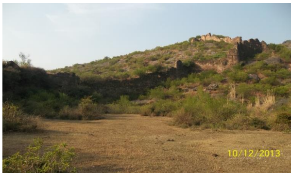
Fig. 3 General view of fortification wall, Pharwala Fort
